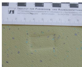
Damage pattern caused by sharp-edged furniture foot
